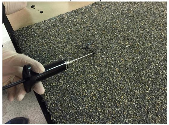
5. Once pressure is relieved, press down plunger to inject BD Patch Coat SC repair material into blister area.
