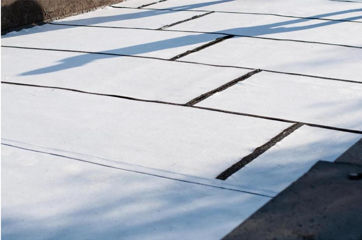
Joints must be sealed using an approved tape (Gerband 602.25). The surface of the SBM mats must be dry during installation of the tape.
