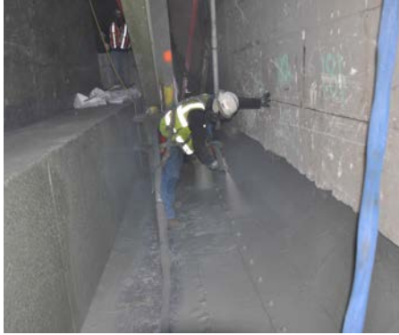
Waterproofing Installation A worker installing Bridge Deck Membrane™ spray applied waterproofing.
