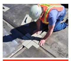
**4-Way Joint** A worker places a 4-way expansion joint at an interesction between the longitudinal and transverse joints.
