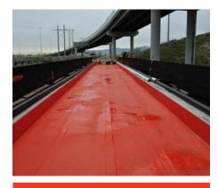
**Completed System** Completion of the spray applied waterproofing on the Winchester bridge.
