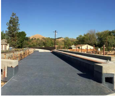
Completed Bridge Deck Completed steel bridge deck with Integrated Ballast Mat.
