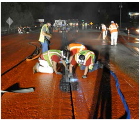
Expansion Joint Installation The Articulus™ Expansion Joint System is sprayed into place using Bridge Preservation™ Joint Adhesive.
