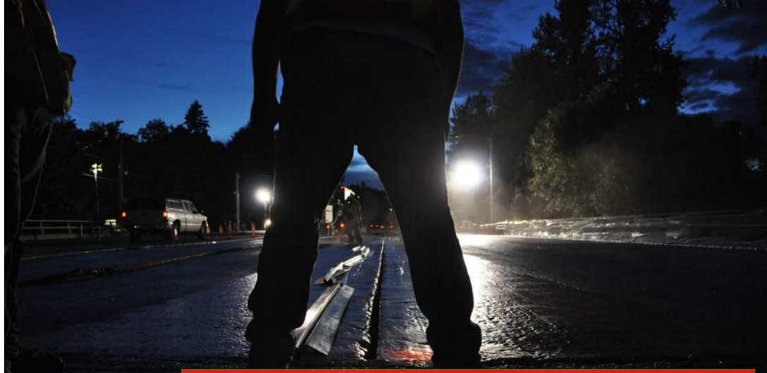
Counter-clockwise from Top Left Surface preparation being performed on bridge deck and joint; application of Bridge Preservation™ BDM; the longitudinal joint prior to the placement of the Bridge Preservation™ Articulus™ Expansion Joint System
