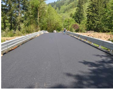
Project Complete The bridge deck is now completely waterproofed and paved.
