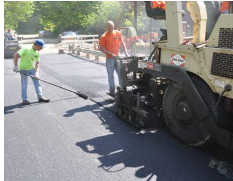
Application of Asphalt The asphalt wear course is applied approximately one hour after the application of the waterproofing membrane.
