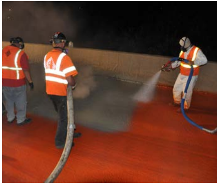
Aggregated Top Coat Aggregate is broadcast into the slower setting top coat.
