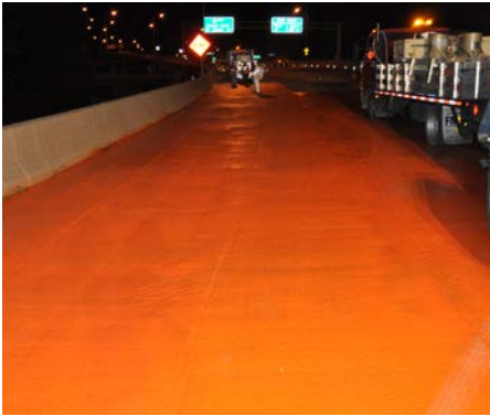
Completed 80 mil System Workers inspect the 80 mil installation prior to the application of the BD Top Coat™.
