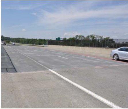
Aggregated Top Coat in Service Aggregated Bridge Preservation™ Top Coat can be used as a temporary driving surface.
