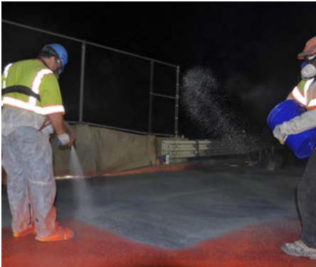
Applying Aggregated Top Coat A worker broadcasts aggregate into the spray applied Top Coat.
