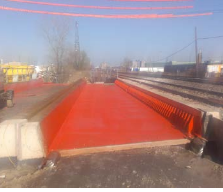
Completed Bridge Detail spray techniques were required to completely waterproof the many stiffener plates on the steel bridge.
