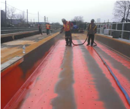
Waterproofing Installation on Steel Bridge Workers install 80 mils of Bridge Deck Membrane™ to the steel surface.
