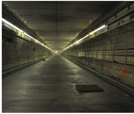
Field Quality Control A Bridge Preservation Technical Representative performing adhesion testing on the newly installed primer.
