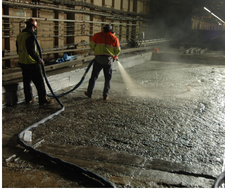
Spray Application Spray application of Bridge Deck Membrane (BDM) to 80 mils.
