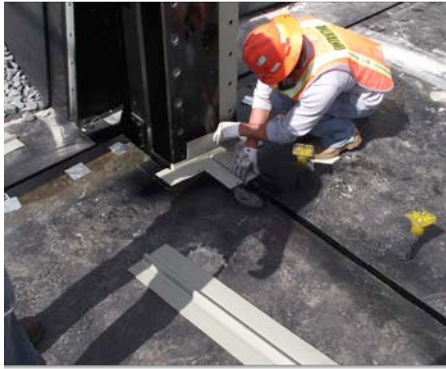
Joint Placement A worker places an Articulus™ Expansion Joint into place
