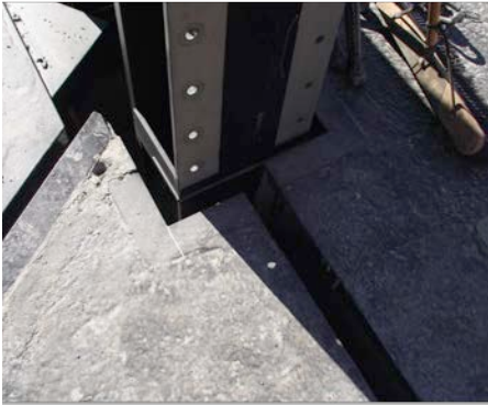
Sharply Skewed Angles Joints with multiple skewed angles that all required waterproofing
